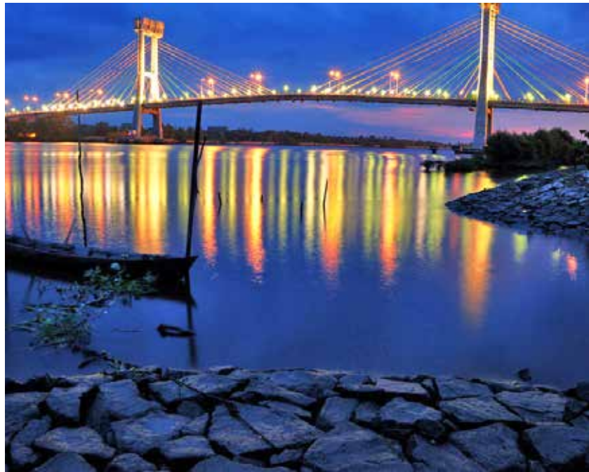
The Tengku Agung Sultanah Latifah Bridge which connecting north side and south side of Siak District was built above the Siak River [Pesona Siak]
